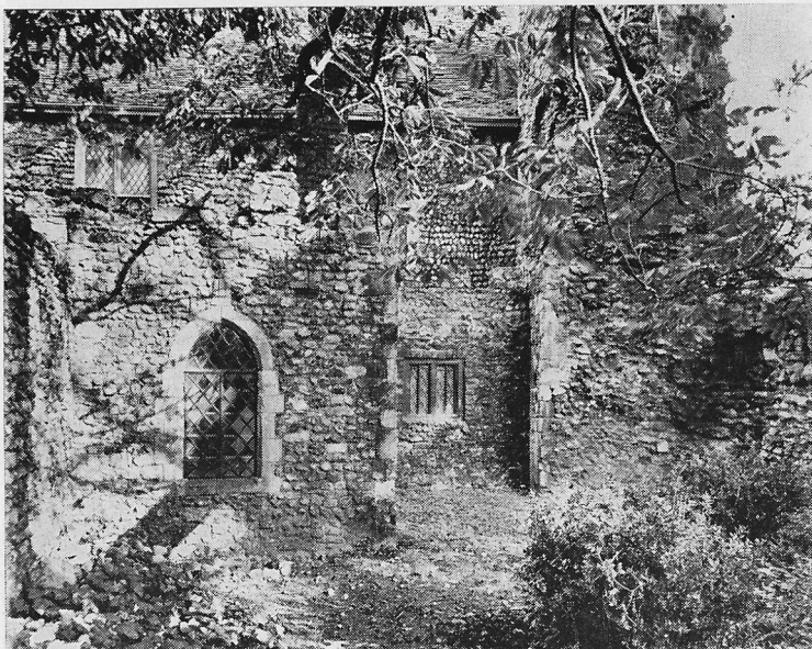
PLATE 3. Minster Abbey: the west front of the west block and tower, showing the varied stone and flintwork, and the fragment of an early window in the tower at gutter level.
