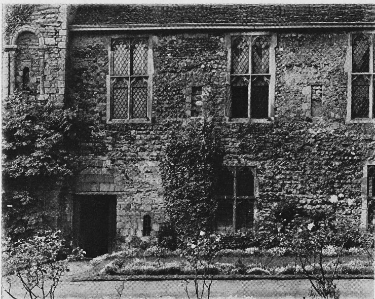
PLATE 2. Minster Abbey: the east side of the west block, with the tower abutment, showing the variations in the wall construction, the Norman doorway, and the original, 12th and 15th century windows.
